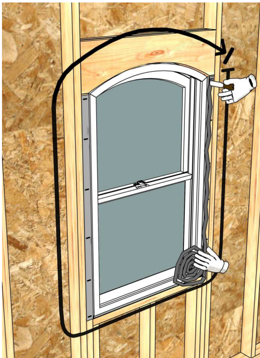
Backer Rod and Sealant Option
