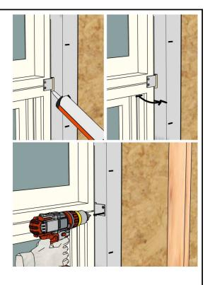
If gusset plates are present, apply sealant between tabs and the opening, bend tabs into position as needed, and fasten tabs as shown. See fastener chart for approved fasteners.
