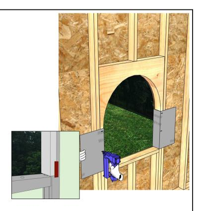
Fold in the house wrap and staple it to the interior of the opening. For steel stud walls, tape house wrap as shown.
