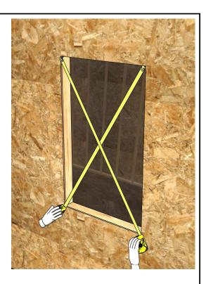
Check that the opening is square. The diagonal measurements should be within 1/8".
