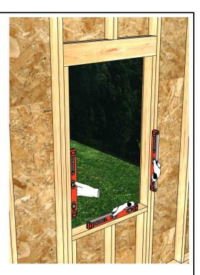
Check that the opening is plumb and level.
